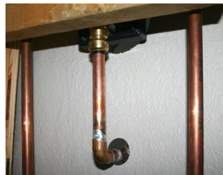
COPPER WATER LINES
