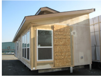
1/2" CCX PLY FOR SITE INSTALLED SIDING
