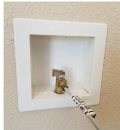
PLUMBING FOR INSTALLED ICEMAKER
