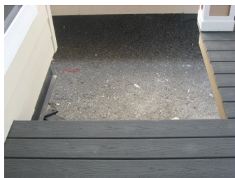
STAIRWAY CUTOUT IN PORCH
