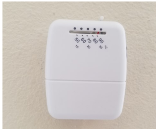
MANUAL HEAT/COOL THERMOSTAT
