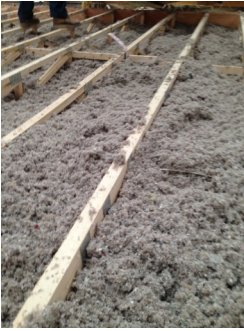
R-22 CELLULOSE ROOF INSULATION
