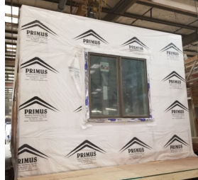
HOUSEWRAP ON EXTERIOR WALLS
