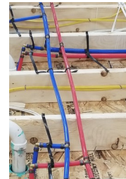
TUFFPEX WATER LINES
