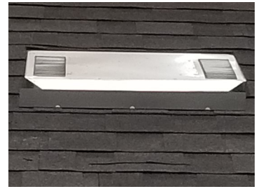
METAL ROOF VENTS
