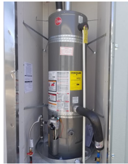
30 GALLON GAS WATER HEATER
