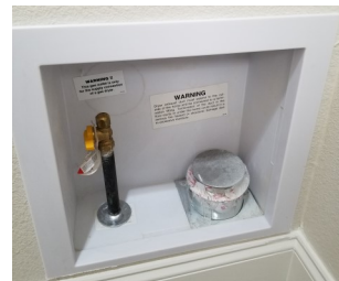
RECESSED WASHER/DRYER PLUMBING
