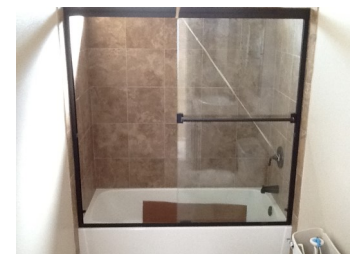
60" TUB ENCLOSURE W/ SURROUNDING TILE
