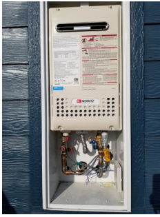
GAS TANKLESS WATER HEATER
