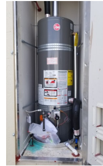
40 GALLON GAS WATER HEATER
