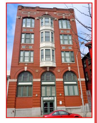
The design of Red Men Hall incorporates a myriad of brick detailing, including brick arches, brick corbeling, brick header trim around tile areas, and a common bond brick pattern throughout the fi-ont elevation, where after every 6th course there is a brick header course. The design also incorporates the use of Indiana limestone and mosaic tiles.
