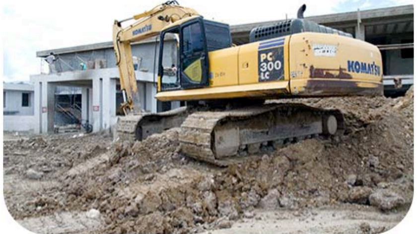
Construction continues on the new Partners In Health hospital in Mirebalais
