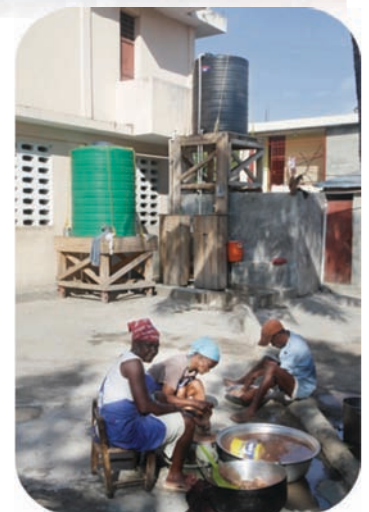
Water purification system at St. Louis School.
