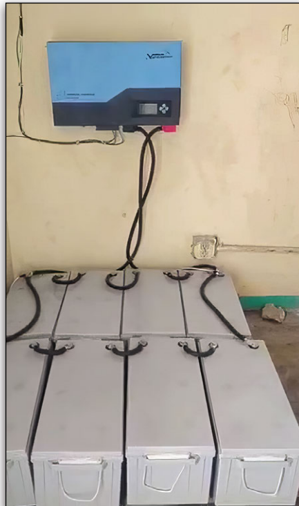
Inverter/Charger and Batteries
