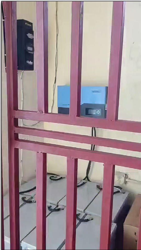
Security Cage for Inverter/Charger, Controller and Batteries
